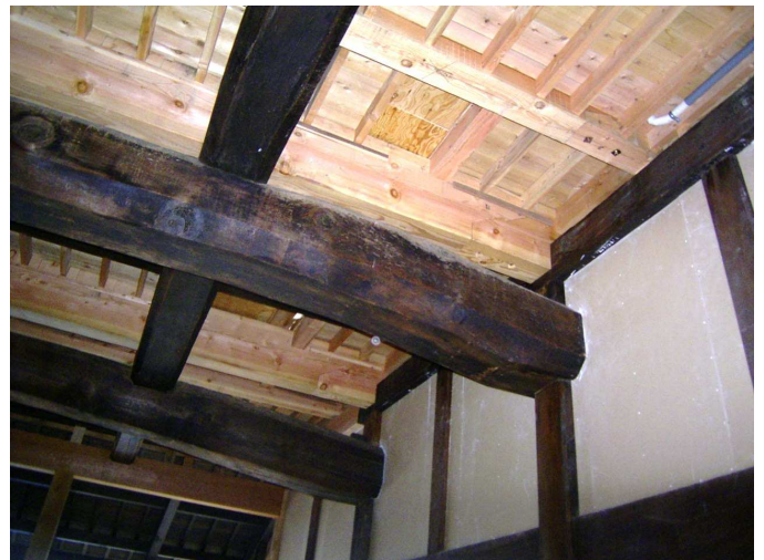
6. 'Dirt floor' beams under construction
